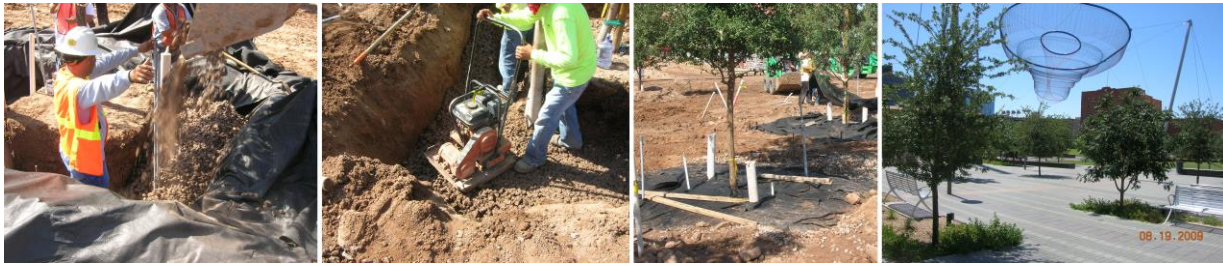
Figure 2. From left to right installation of structural soil and growth of trees in 2009. Images courtesy Richard 'Woody' Dunwoody, Jr.
