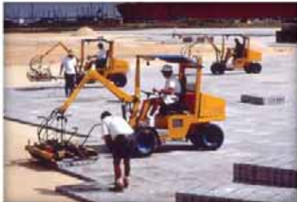
Figure 1. Mechanical installation equipment at Port of Tampa, Florida.
