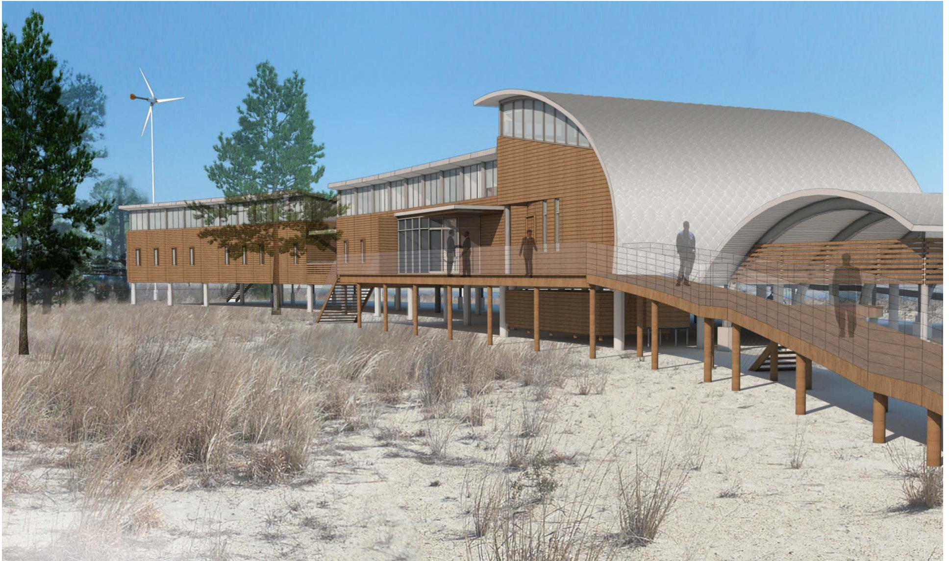
Brock Environmental Center for Chesapeake Bay Foundation, Virginia Beach, VA Targeted Net Zero Energy & Water
