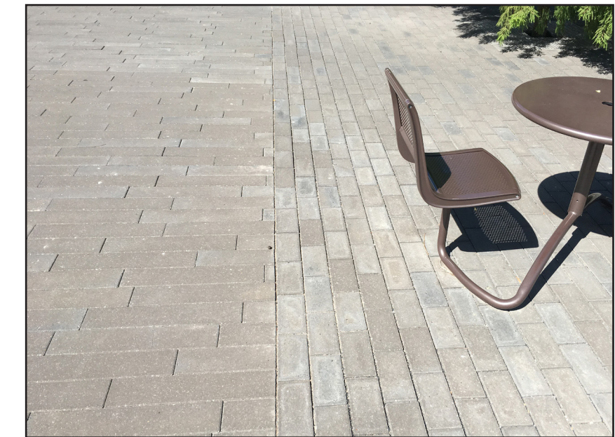
PERSPECTIVE VIEW OF TRANSITION BETWEEN CONCRETE PAVER AND PERMEABLE PAVERS
