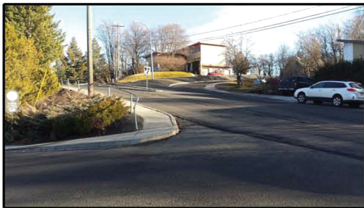
1. Taylor Ave Entry - All water from street flows right onto site
