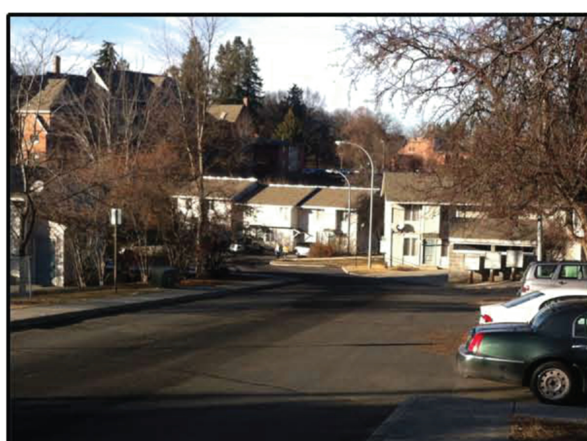
9. Looking in from Taylor Ave. Water flows directly towards buildings, bypassing drains because of poor placement.
